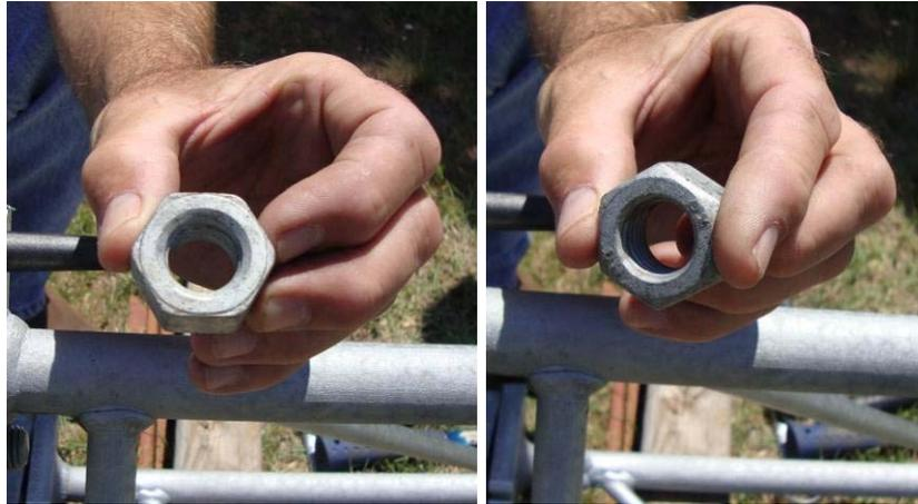
The nut should be applied with the flat side facing the connection (picture on the left). The writing on the nut should face away from the connection.
