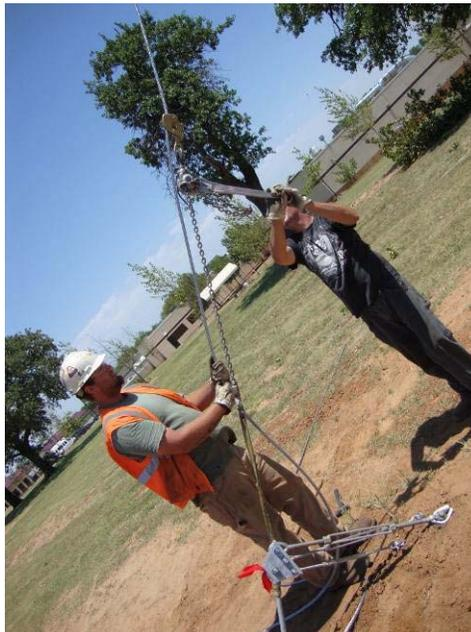
**NOTE:** The 5/8" wire rope used for the top guys in the 140' and 160' towers is very stiff and heavy, making it more difficult to pull the cable and form a proper loop at the
