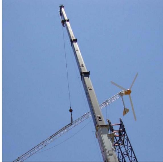
21. Raise the tower/turbine to the vertical position and maneuver it over the base pad. The guy wires may be used as tether lines, but it will be necessary to grasp the base section to align the tower properly on the pier pin.
