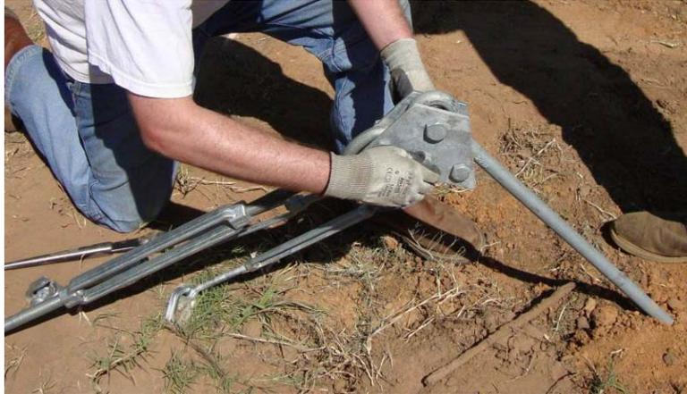
Tighten the 3/4"x3" bolt that goes through the eye of the anchor rod until there is a 1/16" gap between the plates and the anchor rod. This allows the equalizer plates to rotate.
