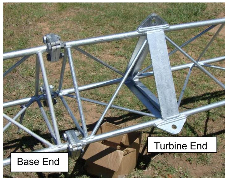
When connecting the top section of the tower, the end with the braced guy tabs will be on the bottom.
