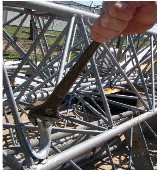
The bigger thimbles for the lower guy cables can most easily be opened by placing the thimble on the tower, resting one side of the thimble along a crossbar. Using a spud wrench, it is easy to pry open the thimble enough to insert the eye connection.
