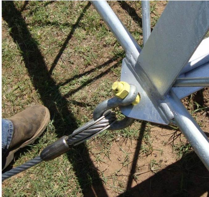
Connect the upper guy cables to the braced guy tabs with the included hardware. Secure the cable with the included nut, and employ a stainless steel cotter pin to retain the nut.
