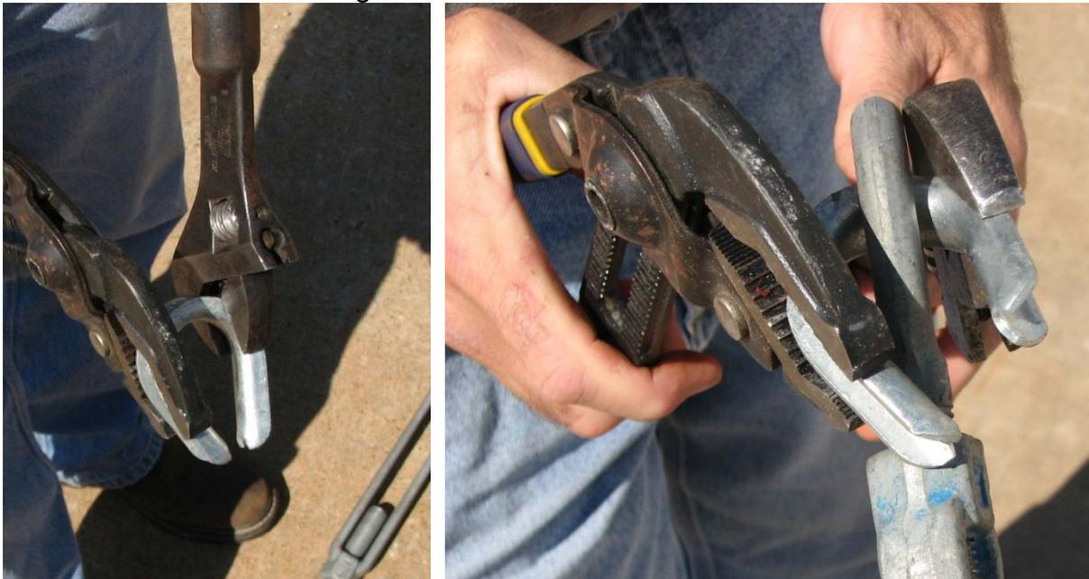
The smaller thimbles can be opened using two wrenches to pry them open. Simply place the eye in the opened thimble and pry it back to the closed position.
