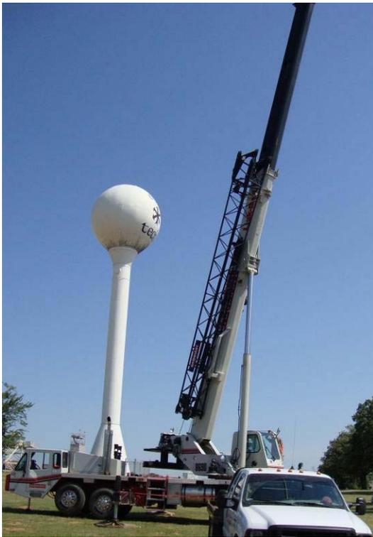
3. Position the crane so it will be **DOWNWIND** of the tower during the lift. (The tail will orient toward the crane boom, keeping the rotor blades away from the cable.) The boom should lean outward to make initial contact with the tower lifting point; boom movement must then be **TOWARD** the crane's center of gravity as the lift and tower placement occurs. (During the lift, the base of the tower will skid across the ground as it moves toward the foundation.)
