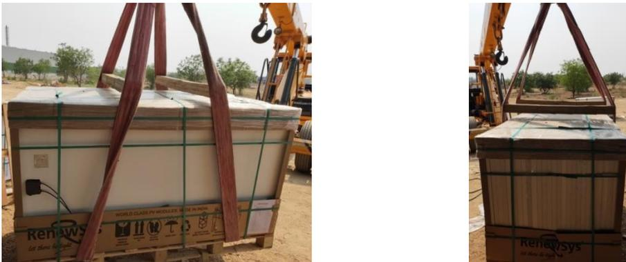
**Fig: Packing Box - Adjusting Sling rope for Hoist Handling
