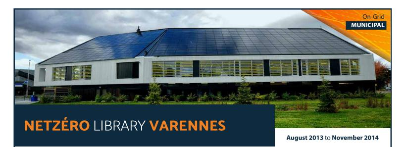
Installation of a 110.5 kW photovoltaic system to supply electricity to the new Varennes Library building
