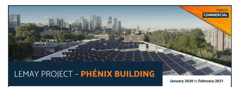
Installation and commissioning of nearly 400 photovoltaic collectors, including 332 bifacial modules, to ensure the production of electricity for the entire office building while contributing to the creation of a zero-carbon building. The panels are also coupled with an energy storage system to serve as an alternate power source in case of a power outage.
