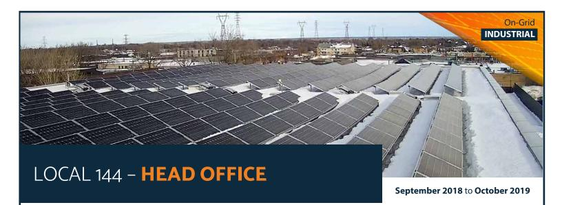
Installation and commissioning of 442 bi-facial solar panels on the roof of Local 144's new headquarters building as part of a large-scale project to create clean energy on an energy-efficient building.
