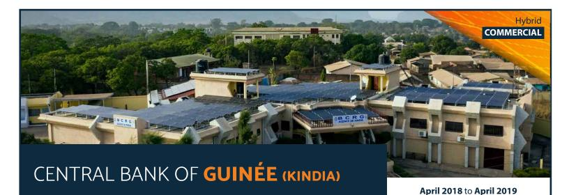
Design and management of a rooftop photovoltaic system -120 kW Design and management of a 120 kWh energy storage system (lithium batteries)
